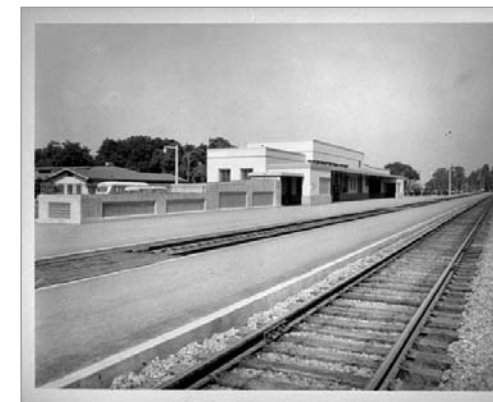
1941 photograph of the newly completed Southern Pacific Train Depot taken next to the north-bound track just south of the station. The Hostess House is visible to the left of the depot. Baggage carts and several automobiles are visible in the parking lot behind the station. El Camino Park can be seen in the distance.
