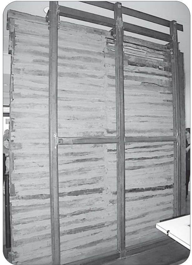
Preserved wall from the rear.
