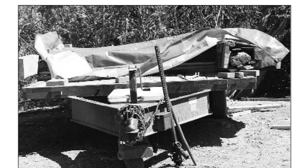
Wall being prepared for relocation and storage at Foothill Park.
